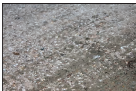
SURFACE FINISH AFTER SCABBLING
