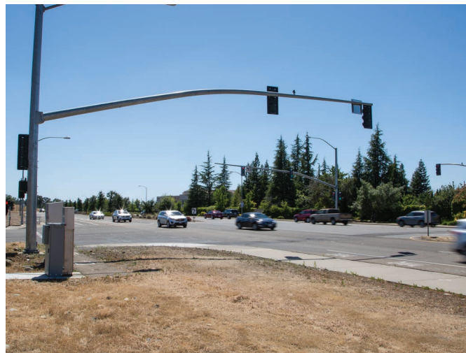
TSP installation, Folsom CA
