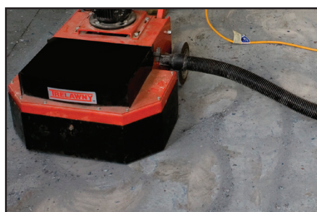
REMOVING HIGH SPOTS
