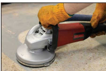
LEVELLING CONCRETE
