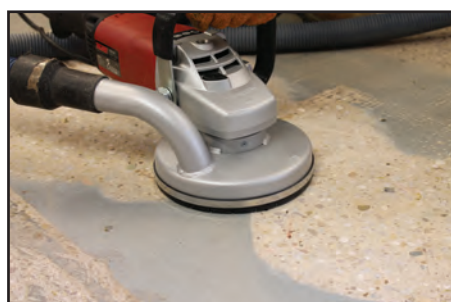
GRINDING CONCRETE
