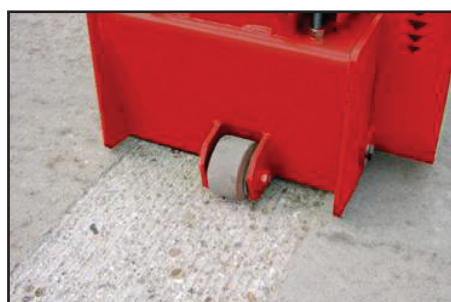
ROUGHENING CONCRETE
