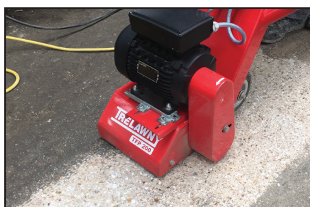
ROUGHENING CONCRETE
