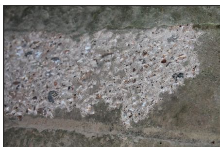
ROUGHENING CONCRETE
